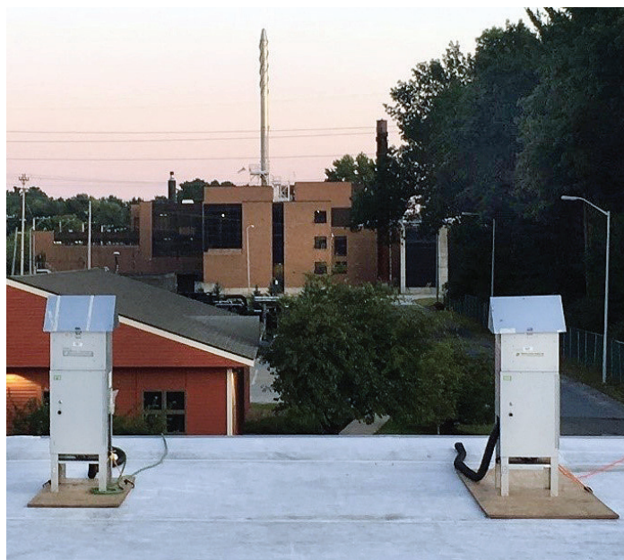
Battelle PFAS Air Insight samplers (foreground) with incinerator stack (background)
