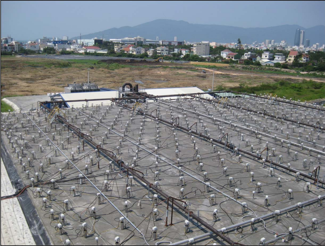
In Pile Thermal Desorption (USAID- Danang Vietnam)
