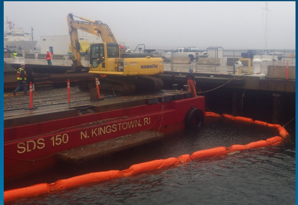
Capping material barge within turbidity curtain
