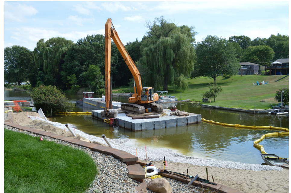
Protection Layer Placement
