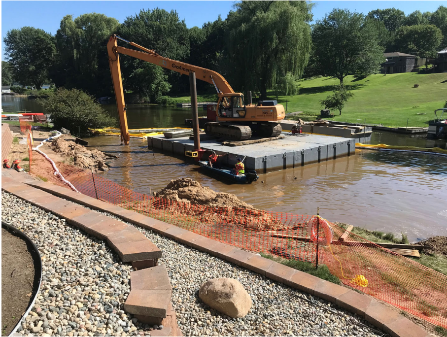
Excavation & Grade Checking
