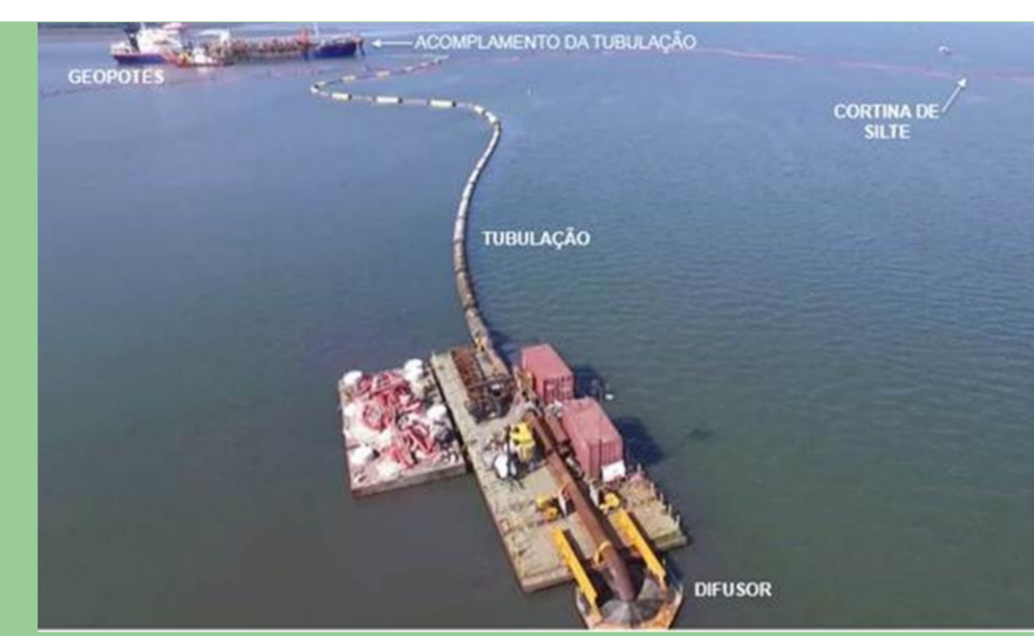
Controls during filling on site
