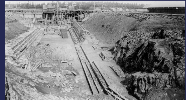
DND Drydock under construction, 1886
