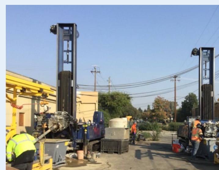
Sonic drill rigs advancing boreholes for injections
