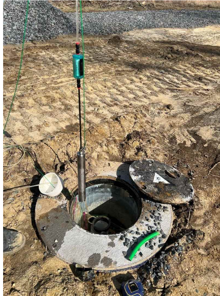
Installation of ISOC Units
