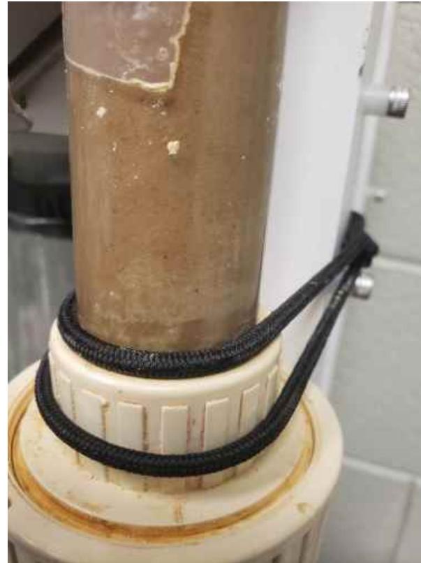
During CLEAN injection and backwashing
