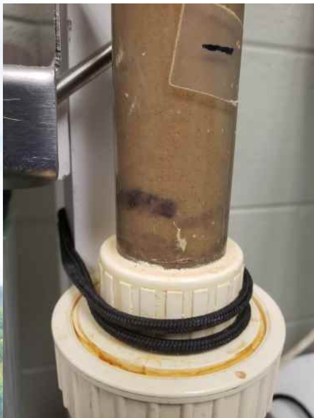
Before CLEAN injection
