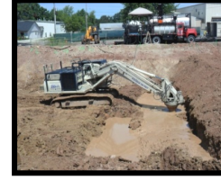
Soil Mixing (Chemical Reagents & Stabilization)
