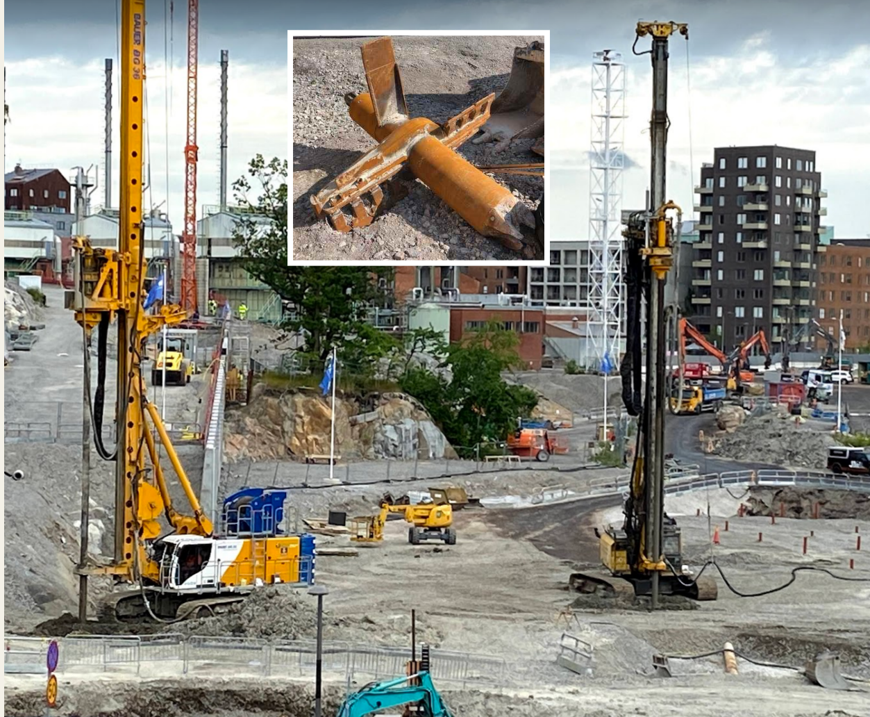
Soil mixing using large diameter augers – 2 rigs in operation
