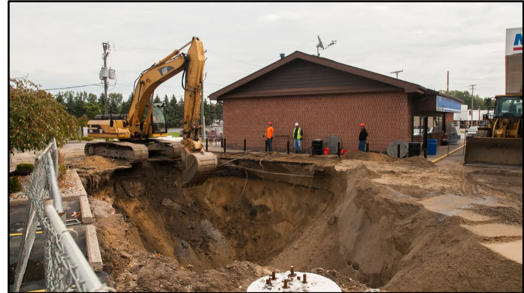
Figure 1: Removal of contaminated soil at a gasoline station by excavation. (Image obtained from: https://www.thetimesherald.com/story/news/local/port-huron/2016/10/17/gas-station-cleaning-up-contamination/92297398/ )
