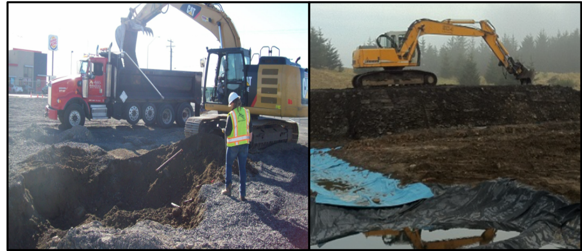
Figure 5: Excavation of a diesel contaminated site and landfill disposal of contaminated soil (Figures obtained from: https://www.ablecleanup.com/portfolio/excavation-of-gasoline-and-diesel/ and https://blog.soilutions.co.uk/2012/08/23/classification-and-disposal-of-contaminated-soil/ )
