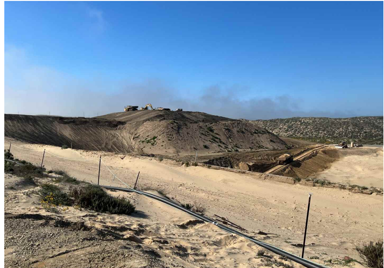
Image 1: Photo of Excavation and Stockpile
